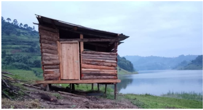
Constructed temporary store/office
